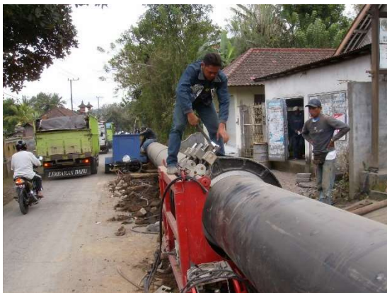
Welding the 800mm OD pipe on the roadside
