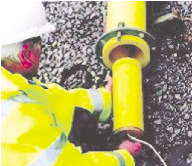
Figure 3: Advanced Pressure Testing using acoustics and creep correction algorithms
