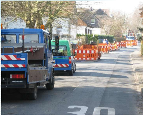
Source: Gelsenwasser AG
