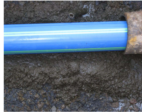
Source: Gelsenwasser AG
