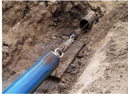
Source: Gelsenwasser AG
