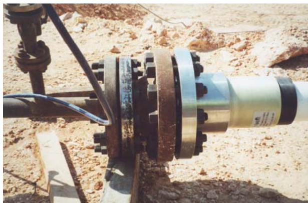
Fig.7 Stainless steel end connection with EF sleeve, Soluforce-Pipelife
