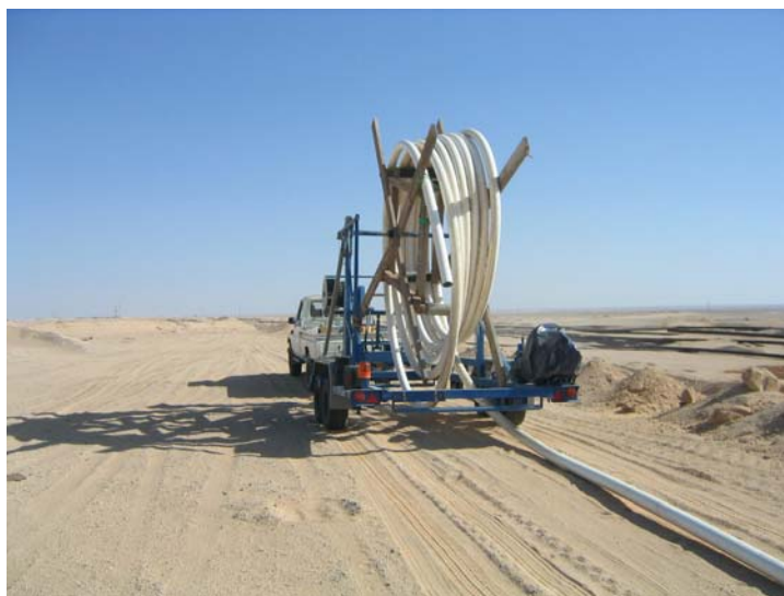
Fig.8 Long length coils avoid frequent joints allowing ‘plough-in’ installation
